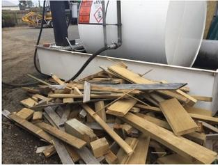
However, recently we have been faced with a number of sites where deliveries have been made unsafe because of either the access to the tank or the stability of the tank. It is important that sites where deliveries occur are free of obstructions and clutter so that drivers are not clambering over things lying around on the ground to reach
