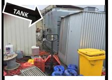
picture reveals just how easy it can be to block the path to a tank on a site. There are numerous items stacked in the thoroughfare that needs to be used to reach the tank, climb the ladder and be able to deliver safely.
